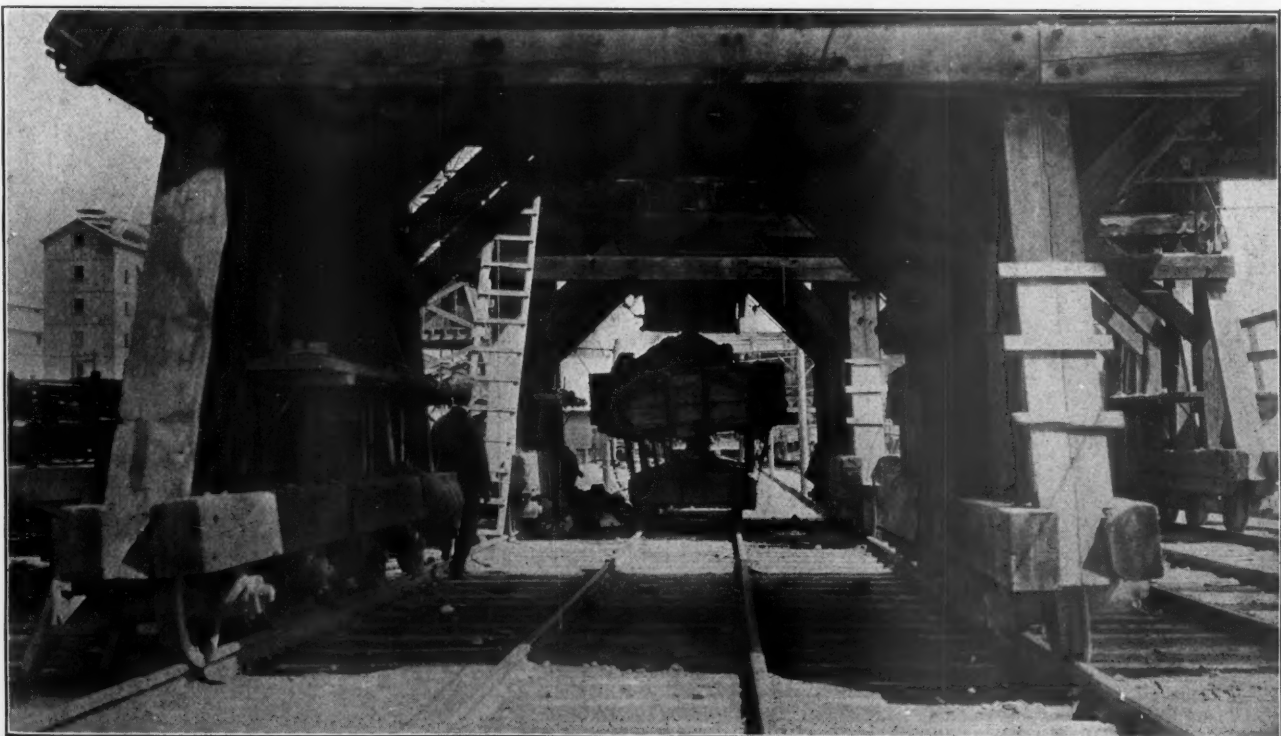
Dump Car Loading Under Rock Bin
